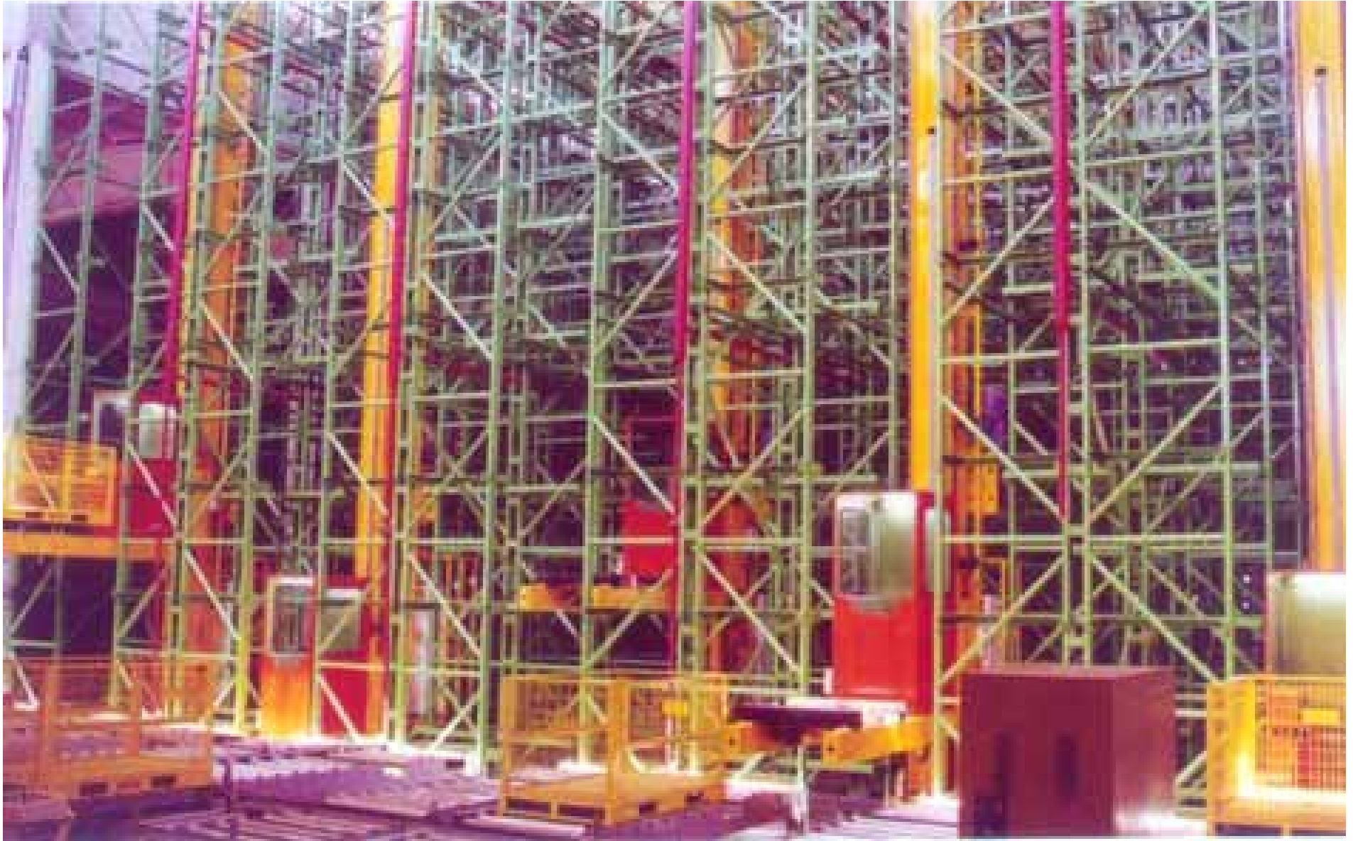
Automated high-rise warehouse, Cargo of Air China
