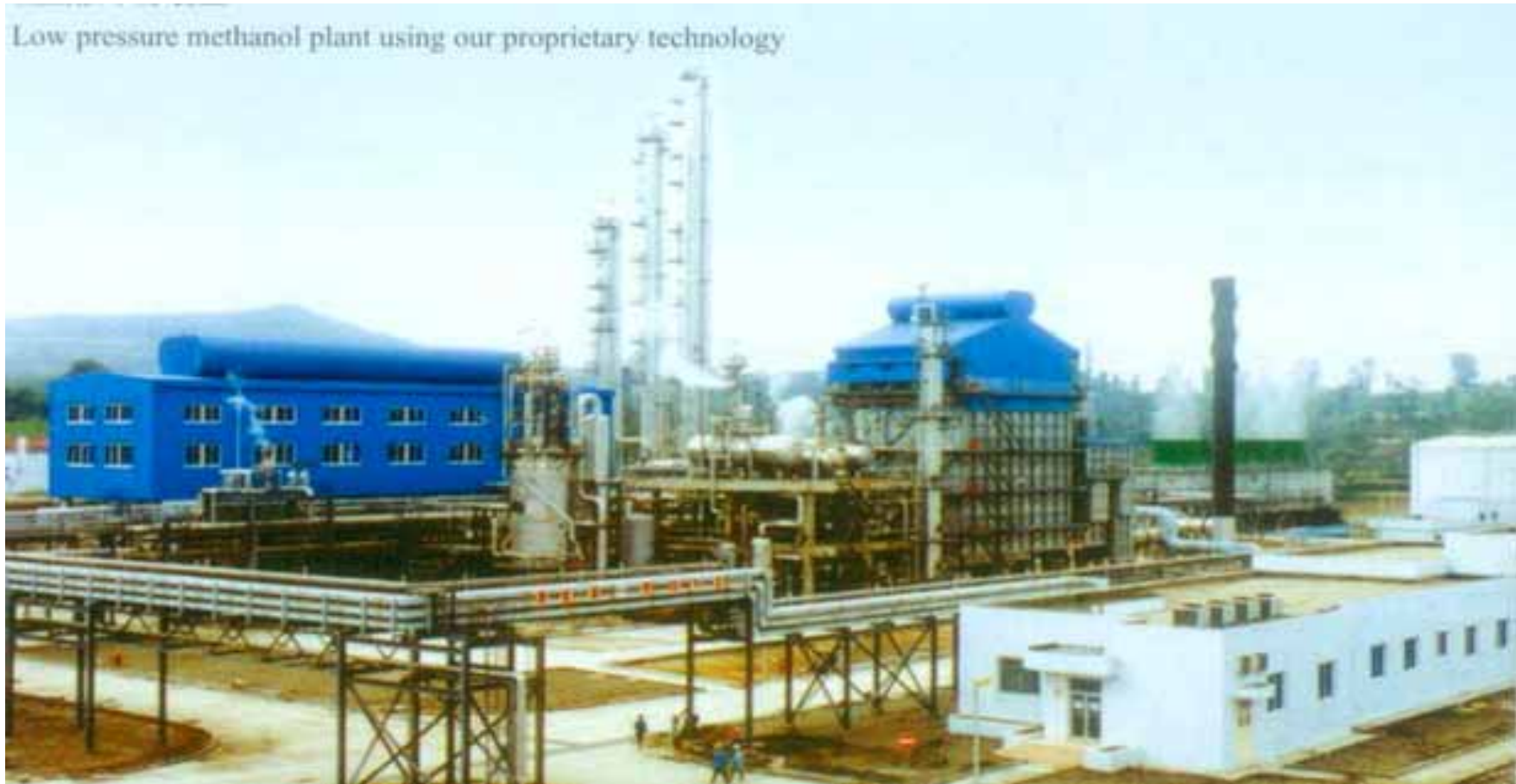
Low pressure methanol plant, China
