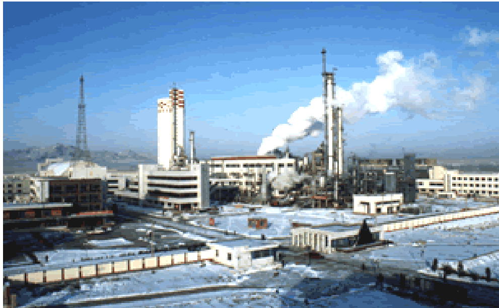
300,000 TPY ammonia and 520,000 TPY urea project of Jinxi Chemical Works, Liaoning, China (1993)
