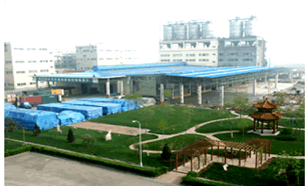
350,000 TPY PVC project of Tianjin LG-DAGU chemical Co., Ltd. Tianjin, China (2003)
