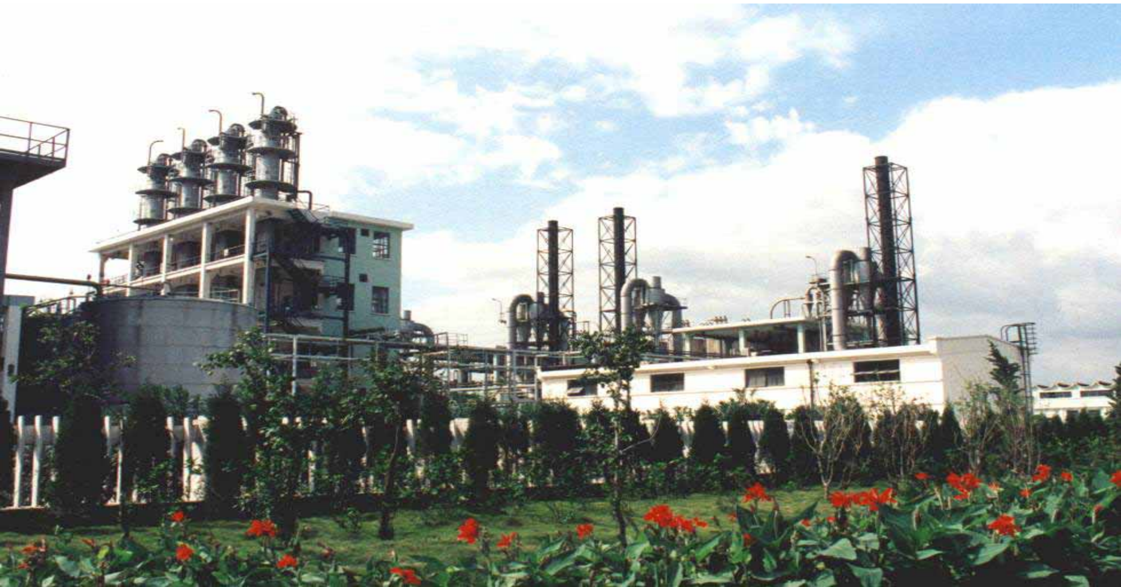
200,000 MTPA VCM Plant, SHANGHAI Petrochemical Corp.
