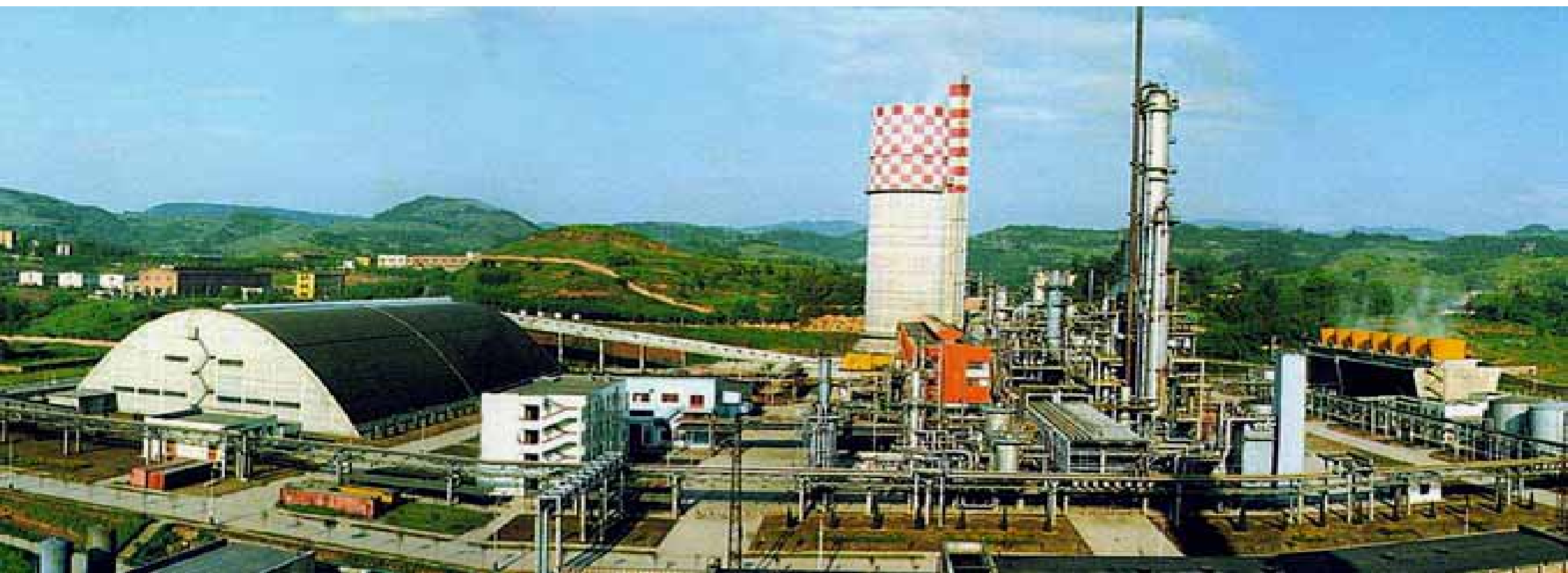
300,000MTPA Ammonia Plant & 520,000MTPA Urea Plant SICHUAN Tianhua Chemical Ltd.
