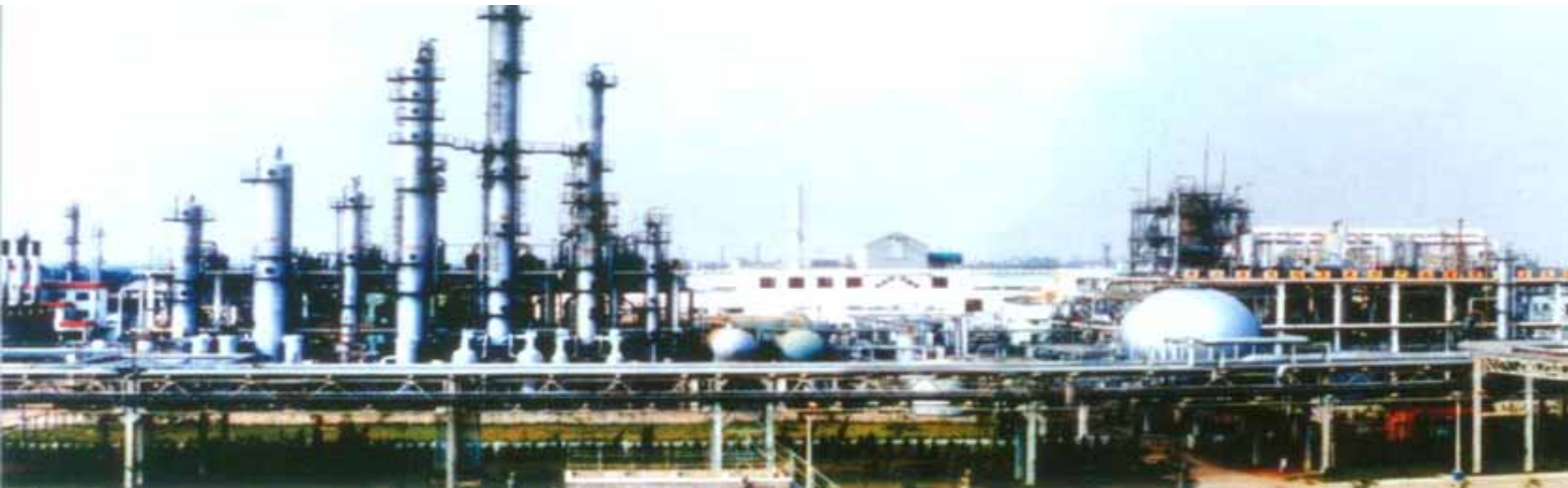
200,000 MTPA VCM Plant, SHANGHAI Petrochemical Corp.
