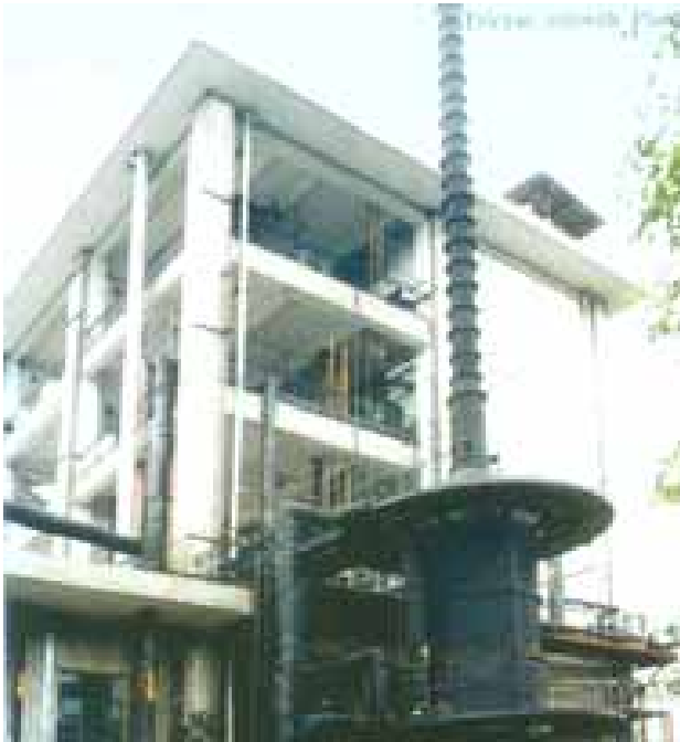
Tricyan chloride plant
