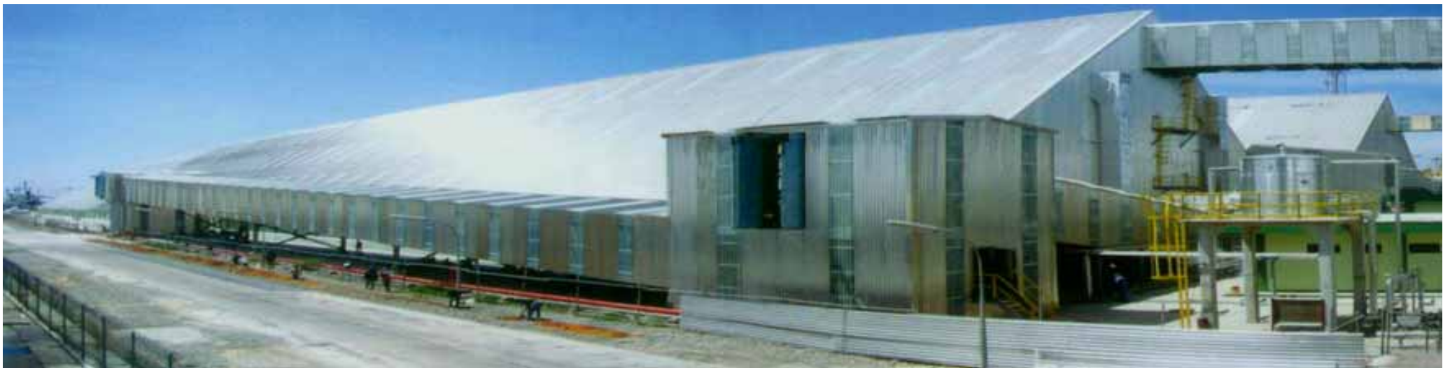
Bulk warehouse and handling system for urea project, Indonesia (2002)
