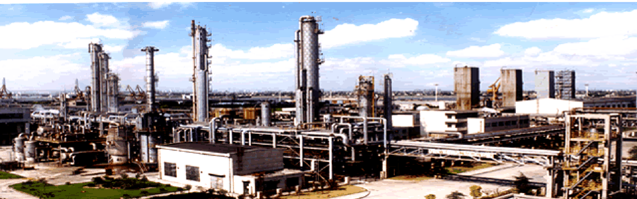
200,000 TPY methanol project of Shanghai Jiaohua Complex, Shanghai, China (1990)
