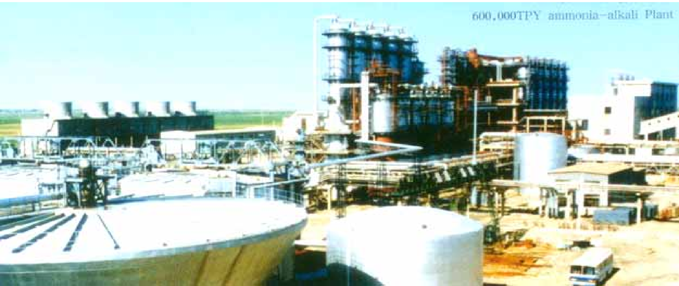
600,000 TPY Ammonia-alkali Plant, China
