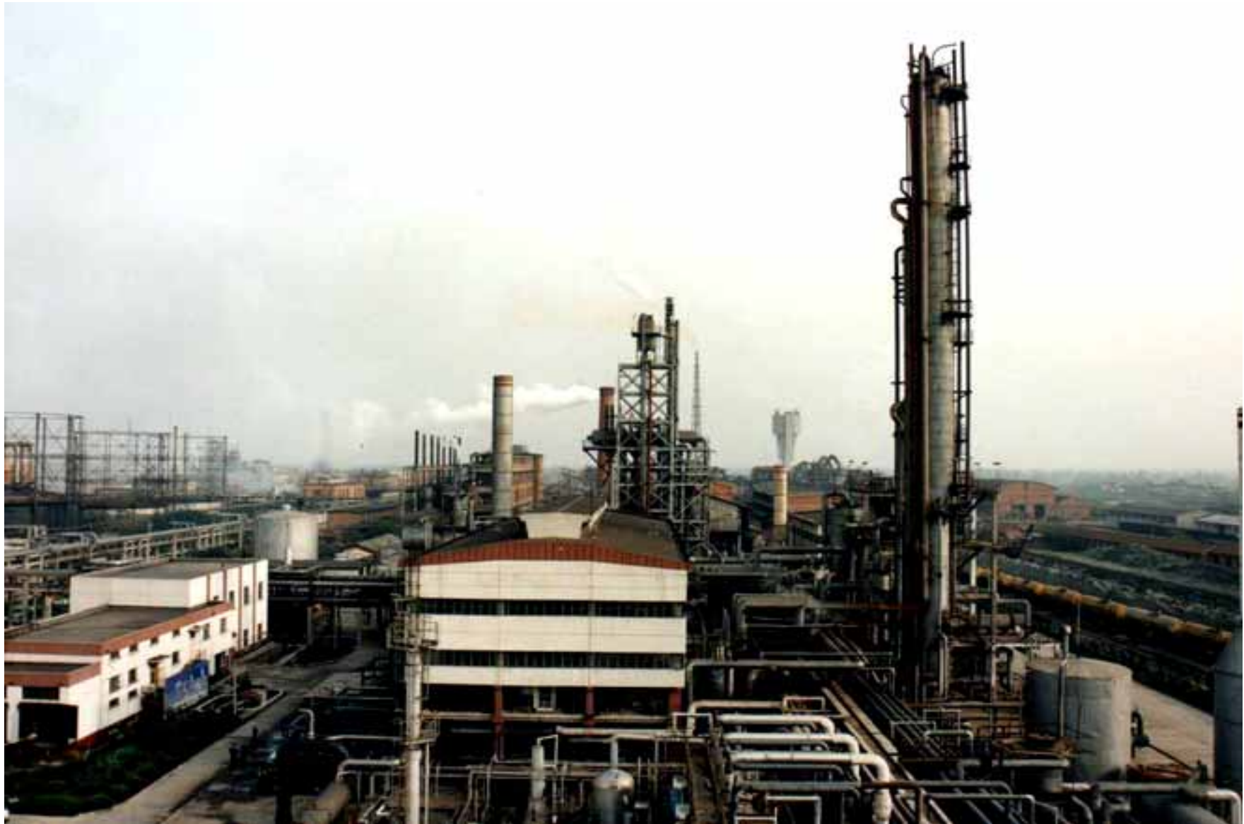
200,000MTPA Ammonia Plant, SICHUAN Chemical Works
