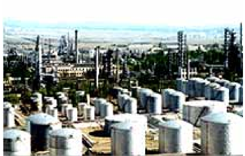
140,000 t/y ethylene project, Xinjiang (1995)
