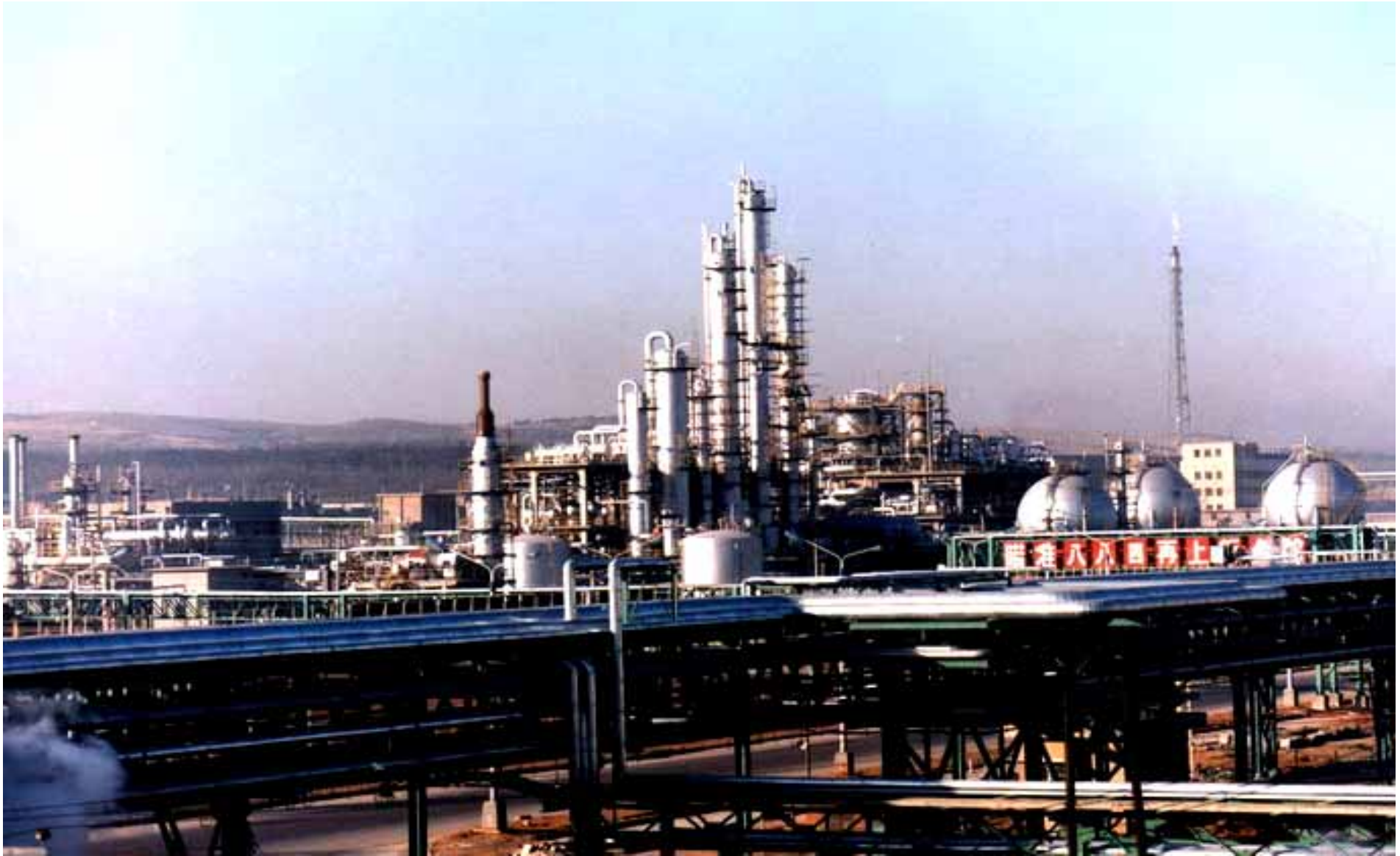
300,000 MTPA VCM Plant, Qilu Petrochemical Complex
