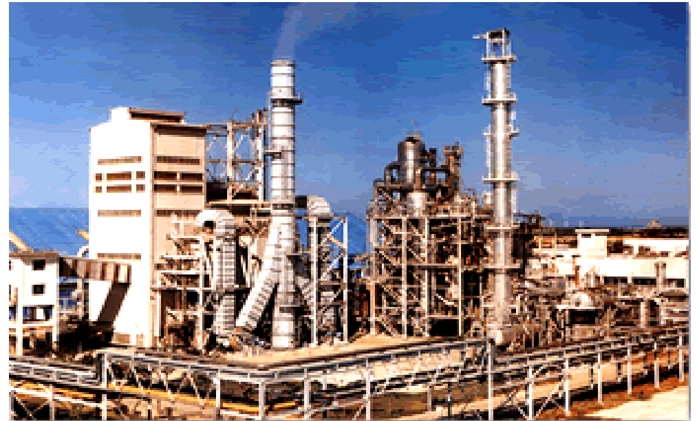
300,000 TPY ammonia and 520,000 TPY urea project of Hainan Natural Gas Chemical Plant, Hainan, China (1996)
