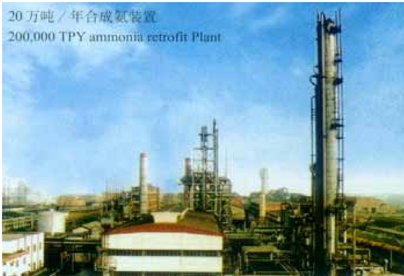
200,000 TPY ammonia retrofit plant, China
