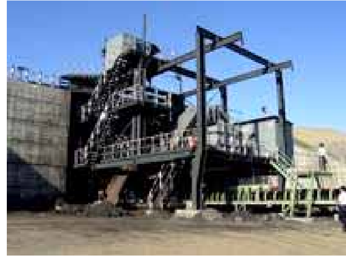
2000t/h Semi-fixed Crushing Station of Huolinhe Surface Coal Mine
