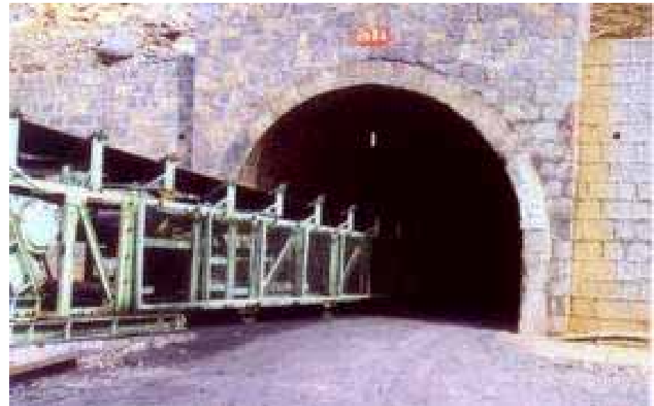
Main incline shaft, Bailongshan coalmine
