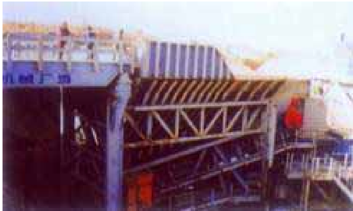
2500t/h Semi-mobile Crushing Station of Haidaigou Surface Coal Mine
