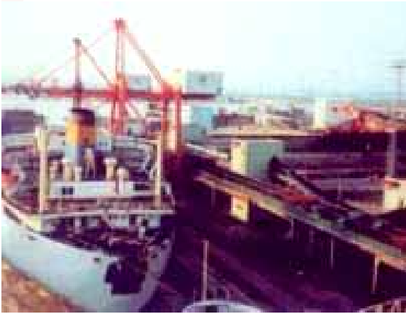
Coal and ore berths, Xinsha terminal, Guangzhou
