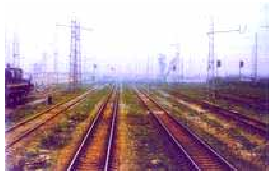
Electrified railway station of surface coalmine
