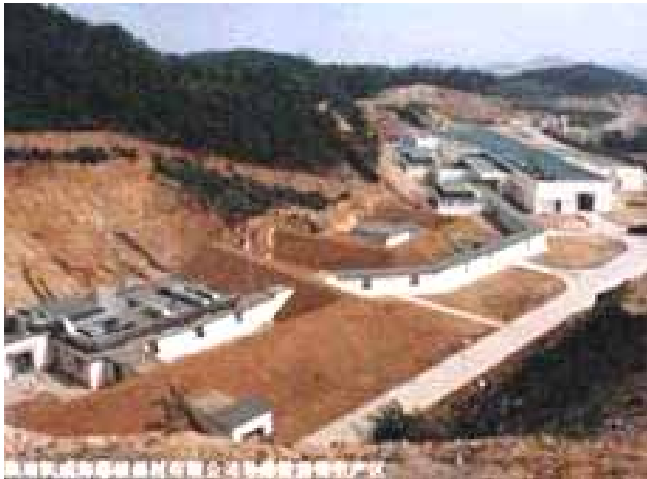
Detonator production section, Auorikai Explosive Products Co, Weihai, Shandong
