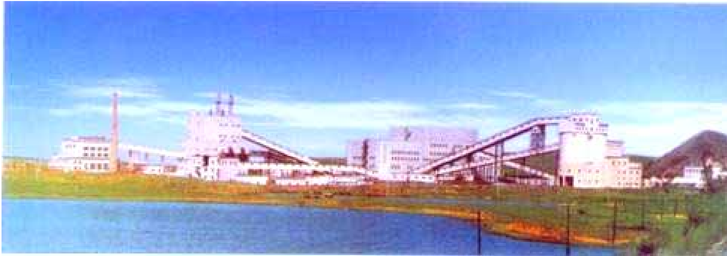
Qixing coal preparation plant, Shuangyashan, Heilongjiang
