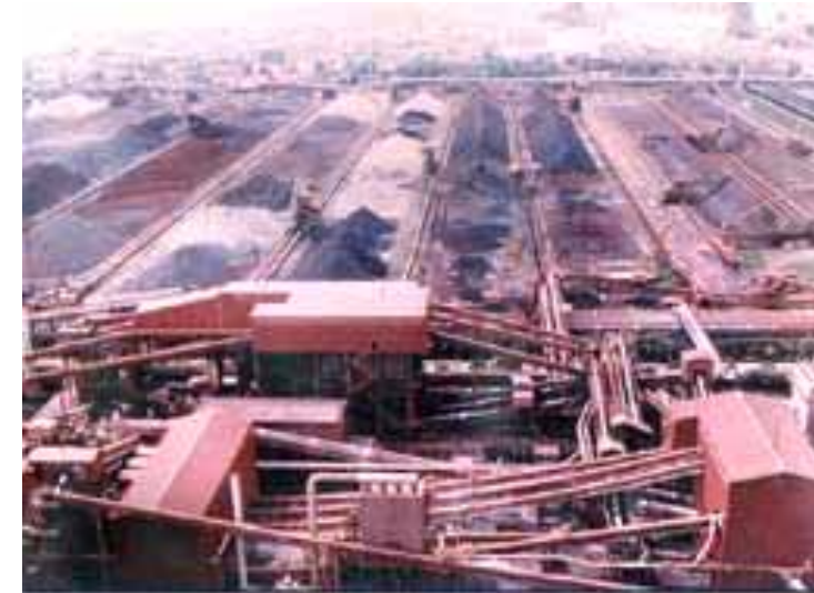
Raw materials stockyard, Phase III, Bao steel
