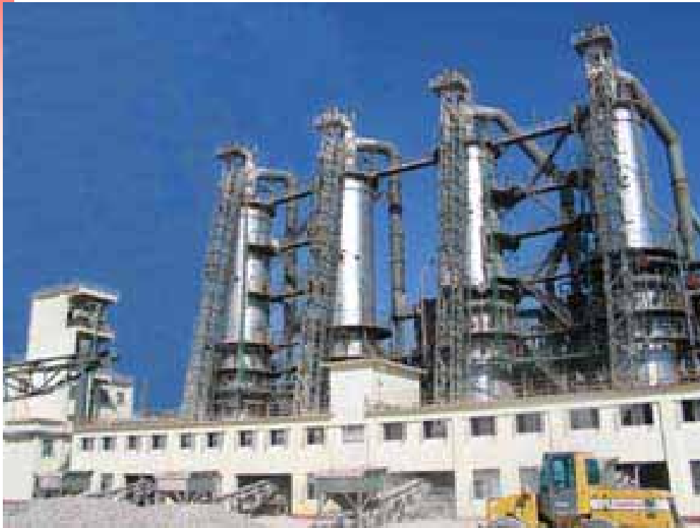
4 x 140 M3 gas burning shaft kiln Shanfeng Group, Tangshan, Hebei (2003.10)
