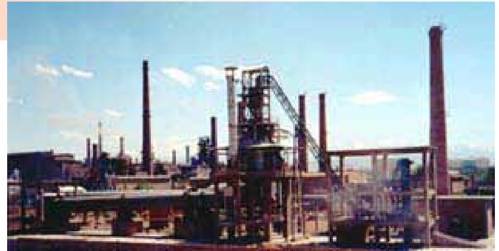
200 t/d, Jiuquan Steel Works
