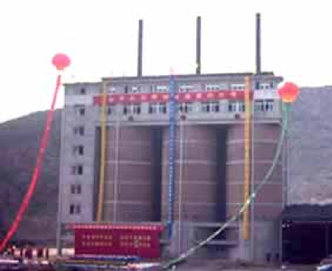
420 t/d, (2nd Phase) Xinghe Building Material Co., Fangshan, Beijing (2003.09)
