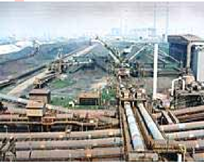
Raw materials stockyard, Phase I&II, Bao steel
