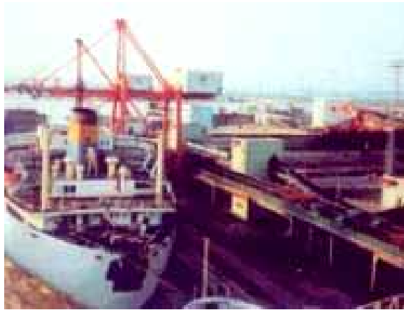
Coal and ore berths, Xinsha terminal, Guangzhou
