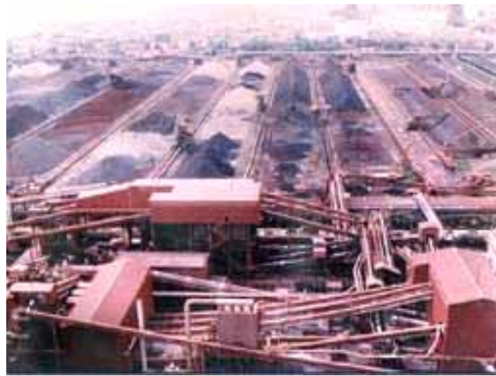
Raw materials stockyard, Phase III, Bao steel
