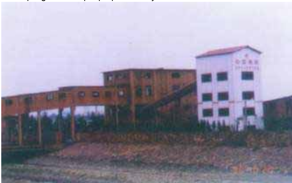
Sampling and sample preparation, belt conveyor carrying and rejecting the sample for mineral terminal
