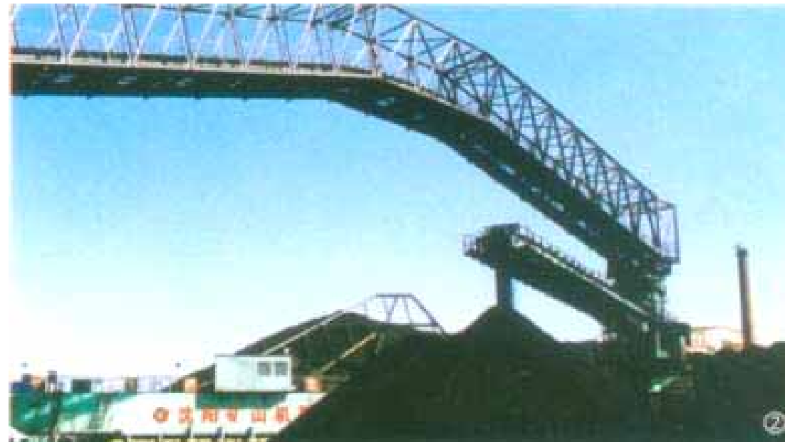
Homogenizing scraper stacker/reclaimer for circular stockyard (outdoor)
