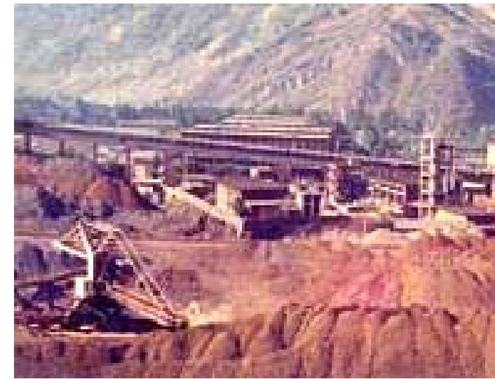
Raw materials stockyard, Penzhihua steel
