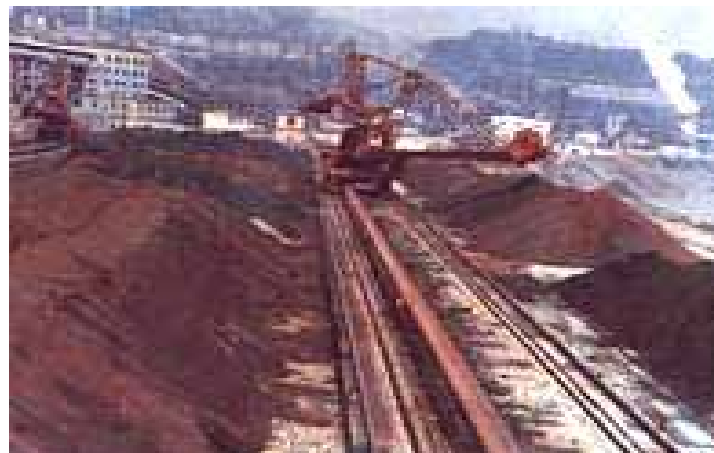
Raw materials stockyard, Chongqing Steel
