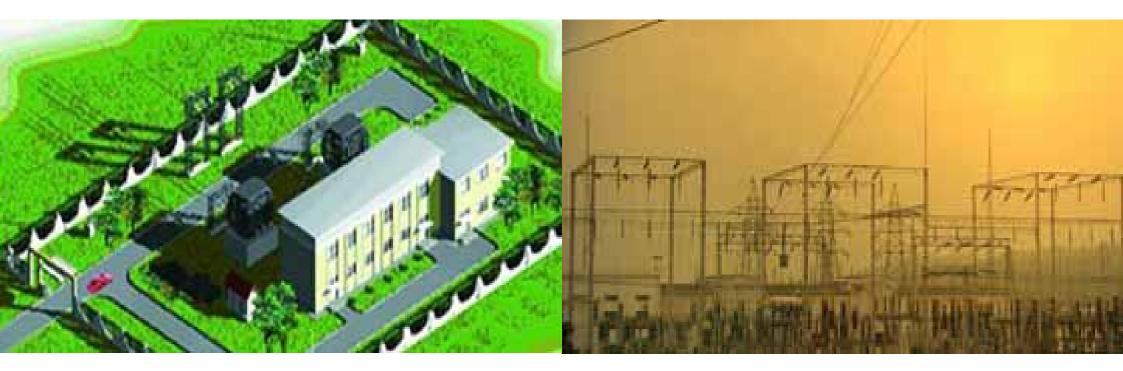
The substation covers Switchgears, Power transformers, Cast Resin type transformers, insulators, Capacitor Bank, SCADA System (Integrated Monitoring, Control & Protection system), and etc.
