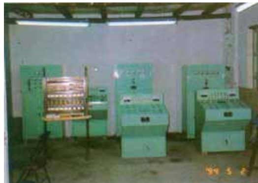
Electric control assembling
