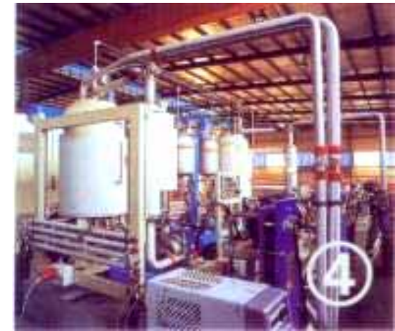
Hi_pressure Metering & Mixing
